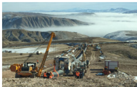
Trans-Anatolian Gas Pipeline (TANAP), Turkey
