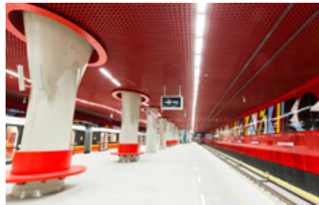
Warsaw Metro Line 2, Poland
