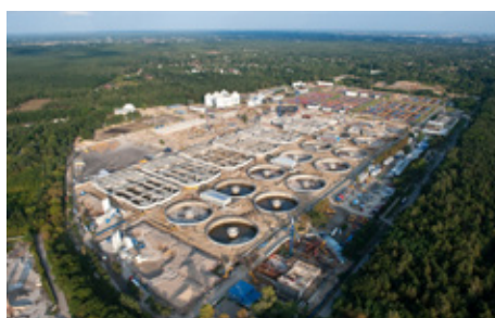
Czajka Wastewater Treatment Plant, Poland
