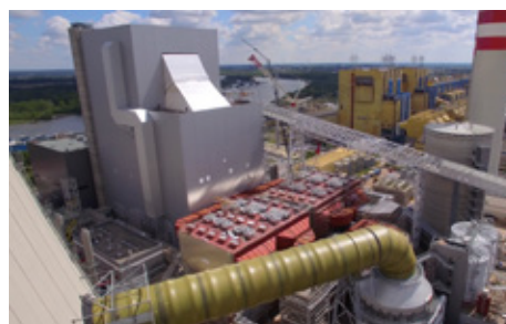
Kozenice Power Plant, Poland
