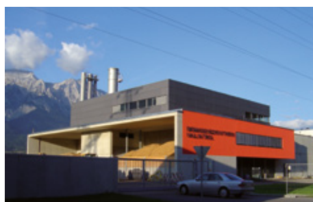
Hall Biomass-Fired Cogeneration Plant, Austria
