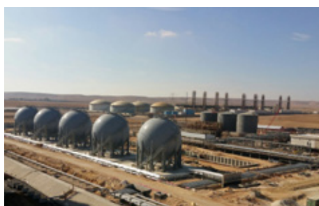
Amman Petroleum Product Terminal, Jordan
